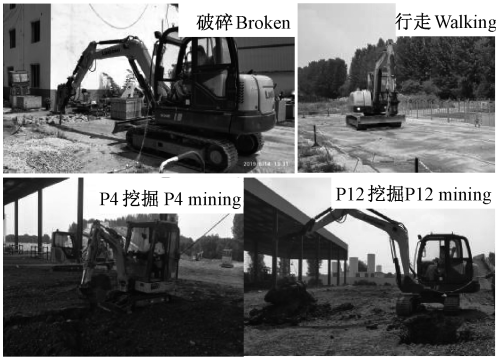
图 4 工况测试 Fig.4 Working condition test
